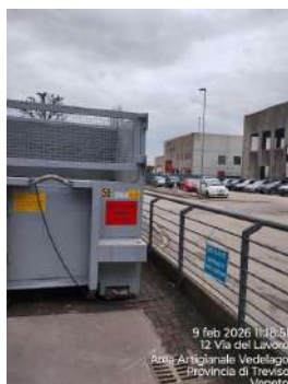
CER code on external waste containers.jpeg
